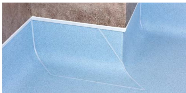
Figure 11 External corners 'wrap around method'
