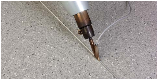
Figure 2 Applying the weld
