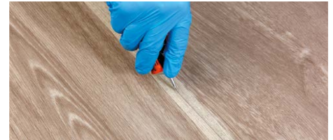
Figure 7 Cold welding
