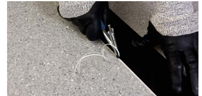
Figure 1 Grooving the seam
