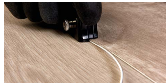
Figure 5 Cutting in the seams
