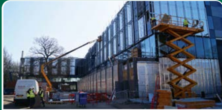
Register as a member to arrange bulk waste collections from your premises or jobsite/projects, saving up to 70%
