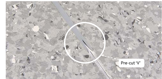
Figure 3 Weld joins
