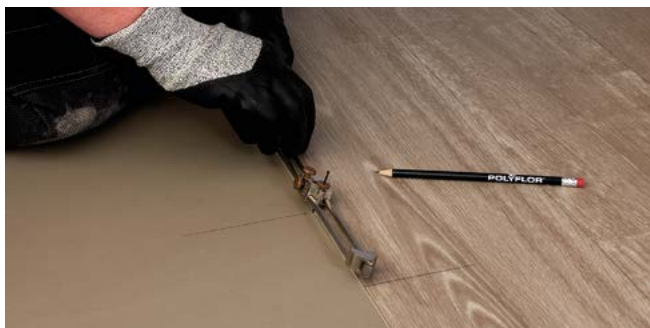
Figure 4 Scribing the wall profile
