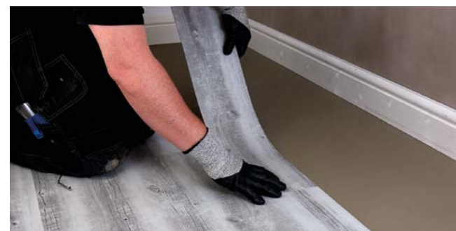
Figure 1 Setting planks out
