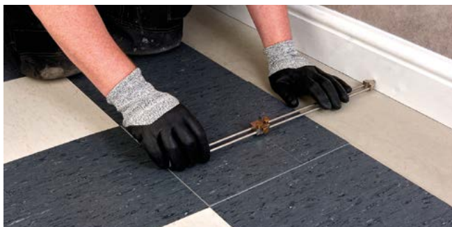
Figure 6 Measuring a tile using a scriber
