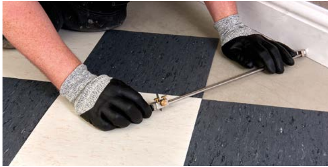
Figure 9 Cutting the tiles using a scribe (diagonal cut)
