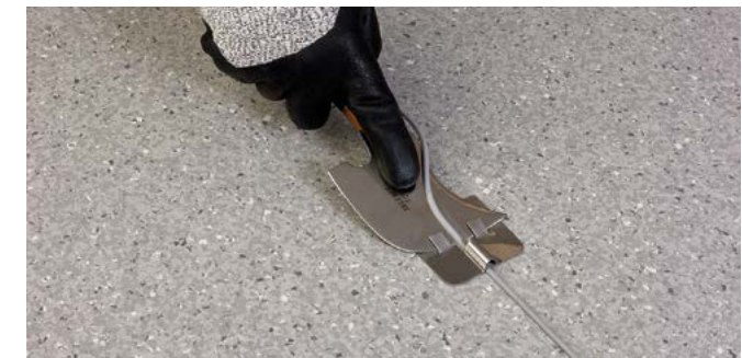
Figure 4a Trimming off the weld top layer (Spatula Trimming Knife)
