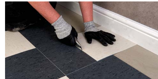
Figure 5 Measuring using an overlapping tile
